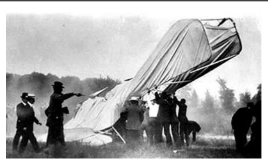
The first demonstration flight fatality in history occurred in 1908 when Lt Thomas Selfridge was killed in this aircraft piloted by Orville Wright. The accident was caused by propeller separation. Orville Wright suffered broken ribs, pelvis and a leg. (17 September, 1908)
